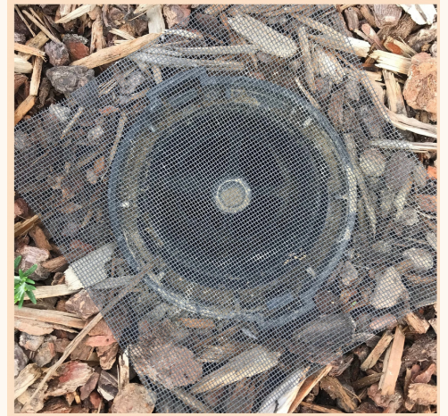
COVER DRAINS WITH FINE MESH
